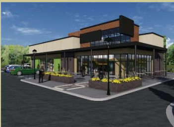
New Structure: Commercial Structure, Wall, NJ
